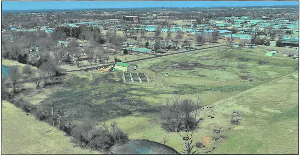
Bethel Heights' Lincoln Street Sewage Dump. Sewage Flooding and Runoff onto Neighboring Property and into the Illinois River Watershed. January 2019 (Joe Brooks)
